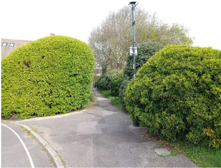
(Above) Existing evergreens at junction of Grove Pastures which enclose the footpath and restrict views of Grove Gardens, reducing passive surveillance and increasing opportunities for anti-social behaviour.
