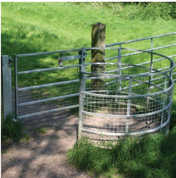
Figure 6 – Proposed accessible RADAR kissing gates to replace existing gates
